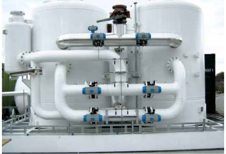
Figure 19: PSA (pressure swing adsorption); ADSOSS®.
