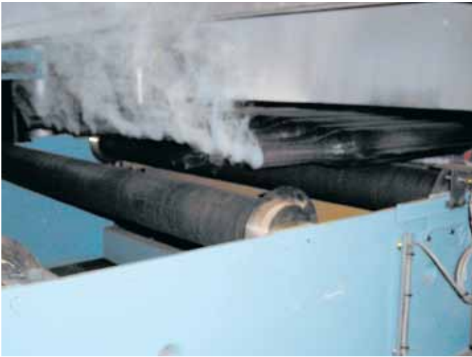
Figure 41: Oil vapours exiting the tube ends at the inlet of a furnace.
