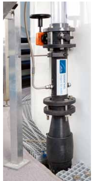
SOLVOX® venturi installation
