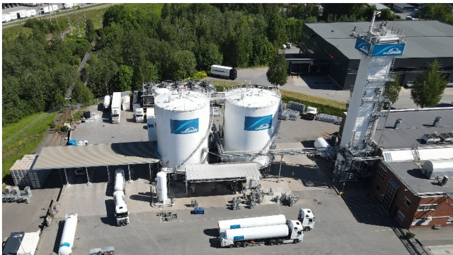
Production plant for air gases: Oxygen, Nitrogen and Argon.
