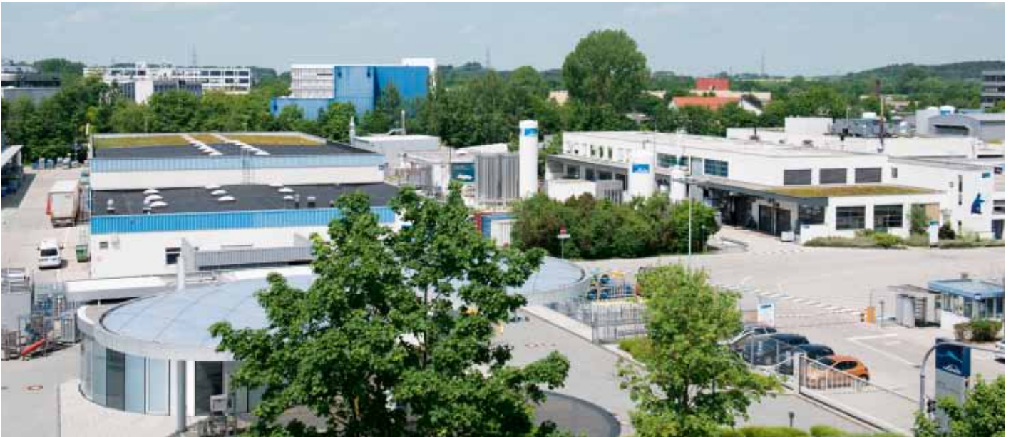
Linde Gas Research Centre Unterschleissheim, Germany.
