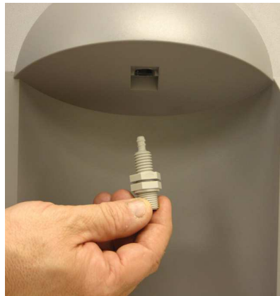
FIGURE I: REMOVING THE DISS FITTING
