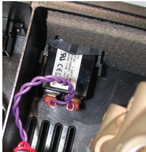
FIGURE AJ: INTERNAL VIEW OF HOUR METER
