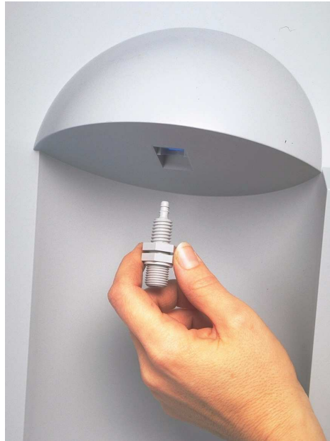
FIGURE M: REMOVING THE DISS FITTING
