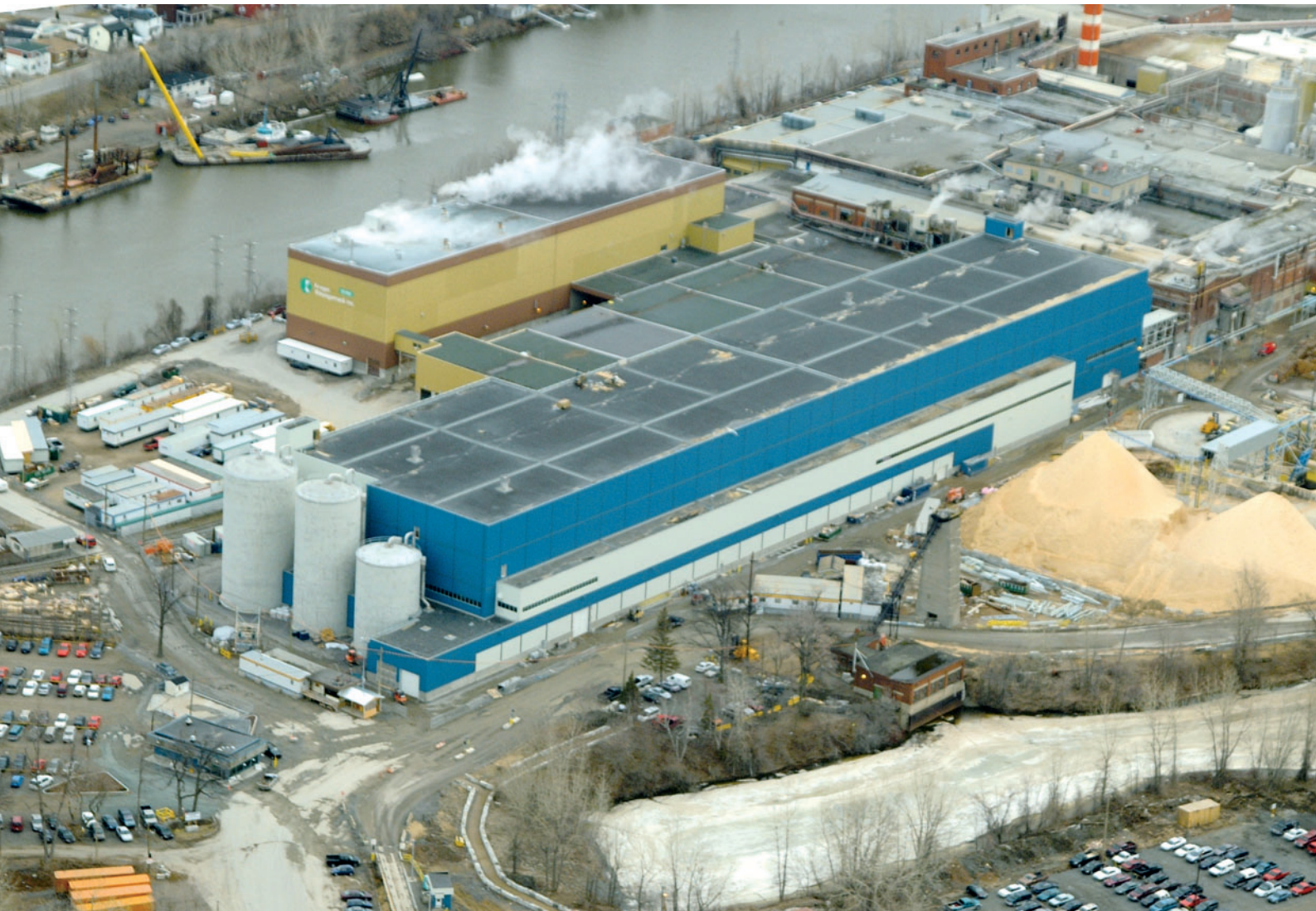
The Kruger Wayagamack paper mill in Trois Rivières, Quebec, Canada.
